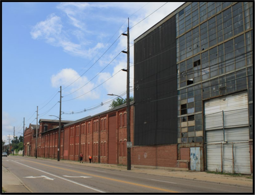
Figure 6 – Looking SW along N. Third St./MLK Blvd.
