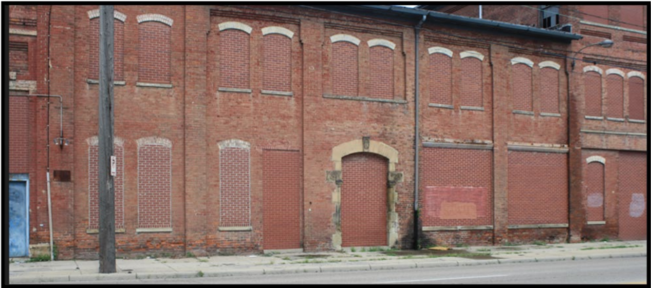
Photo 4 – Looking W along N. Third St./MLK Blvd.
