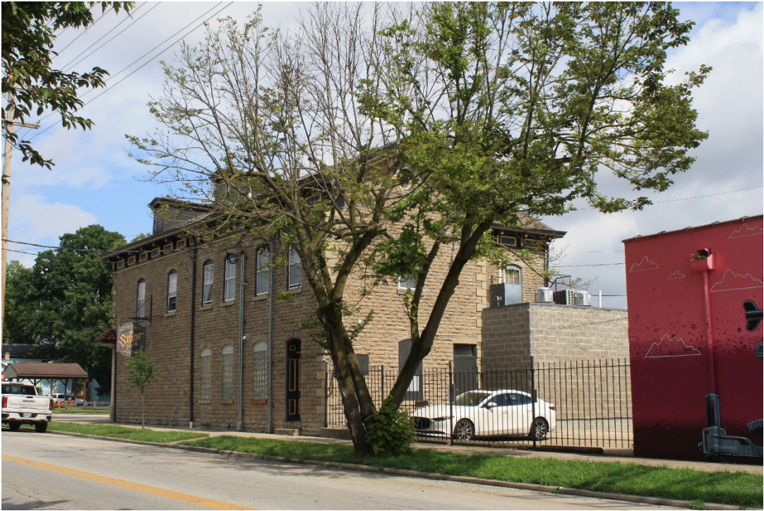
Photo 4: View of Stone Tavern, 701 Greenwood Ave looking Northwest on Heaton St.
