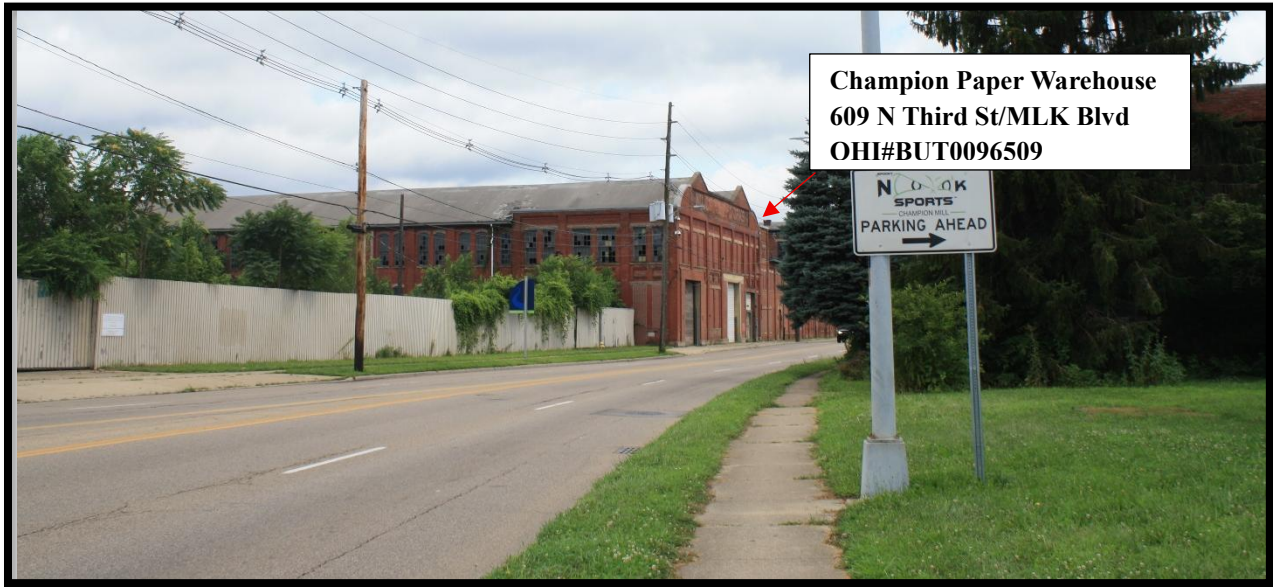
Photos 5 & 6 – Looking NW at West Side of N Third St/MLK Blvd
