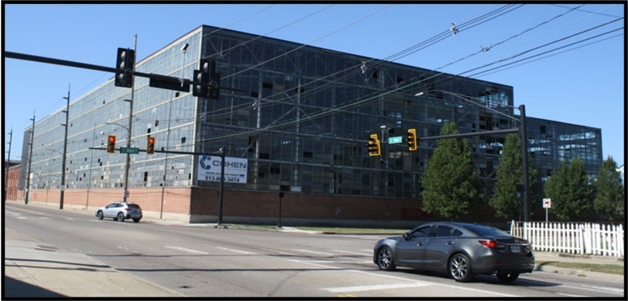
Photo 7 – Looking SW towards intersection of N. Third St./MLK Blvd. & Black Street
