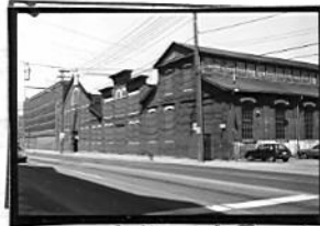
NEC Mill and Third Sts. Niles Tool Works.
