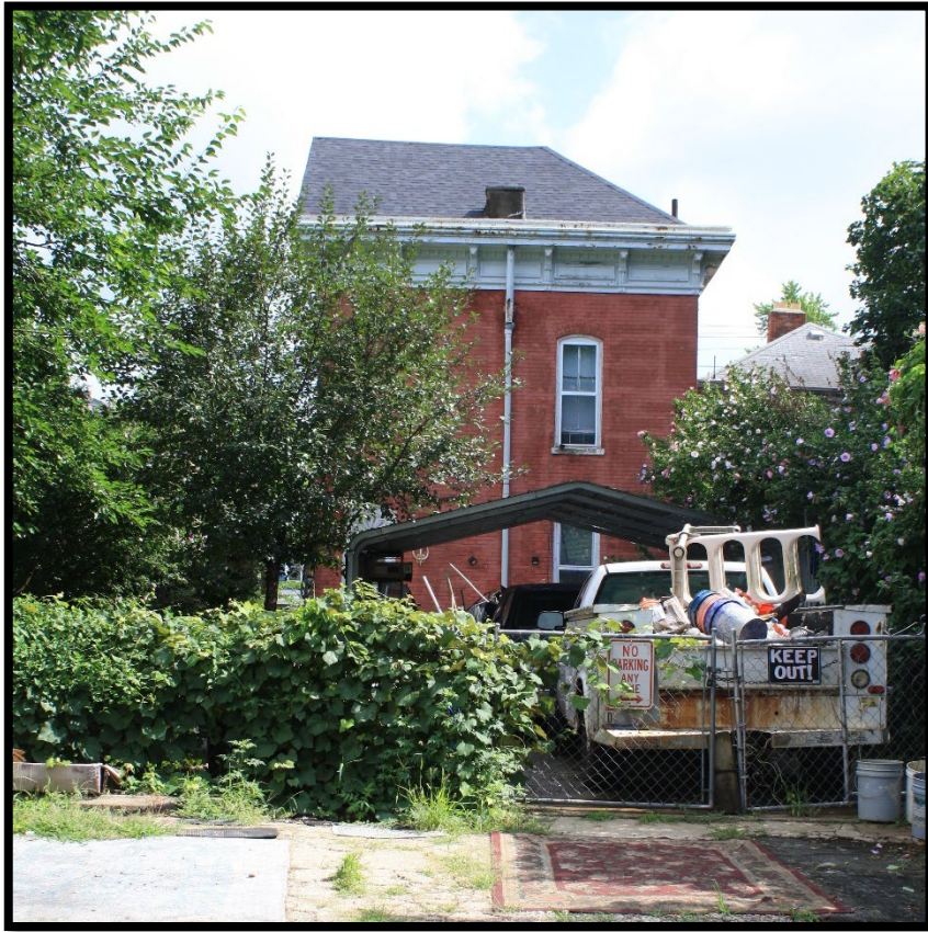
Photo 6 – Looking NE at the rear elevation of 905 Heaton street.
