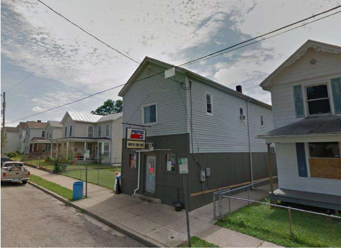
Figure 25: View of North End Market (Google Streetview)
