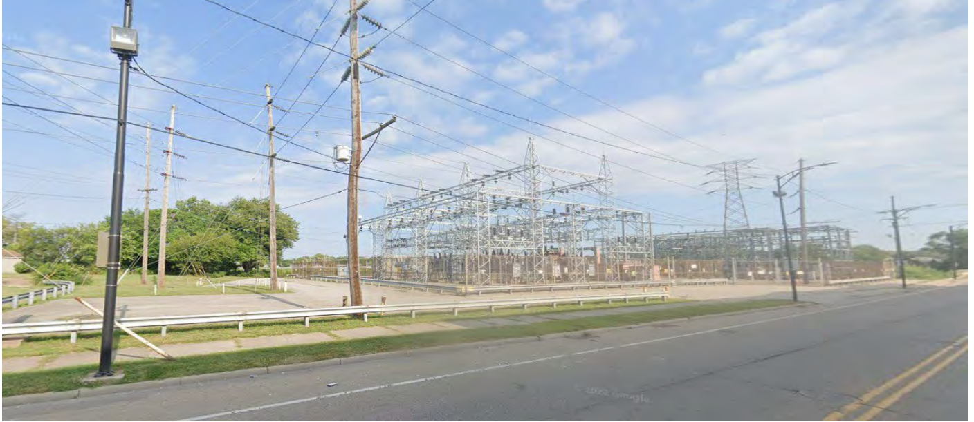
Photograph 3: Site RM-W19. Viewing Power Plant, looking northeast.
