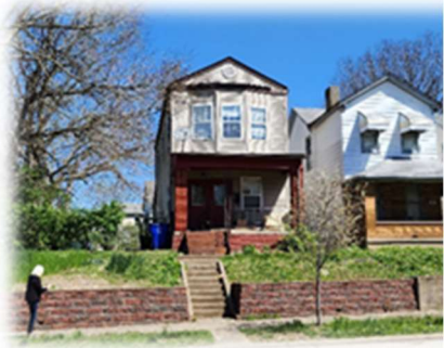
932 Heaton Street P6431025000068 Residential
