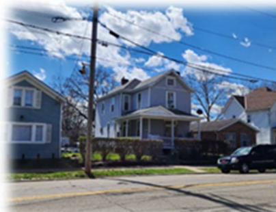
1029 Heaton Street P6431035000010 Residential – Two-Family
