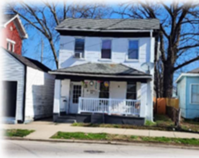
652 Heaton Street P6431017000045 Residential
