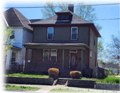
1015 Heaton Street P6431035000006 Residential
