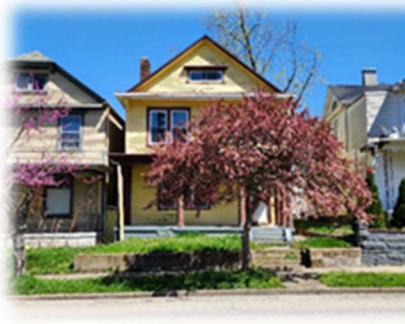
916 Heaton Street P6431025000064 Residential
