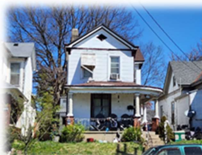
938 Heaton Street P6431025000071 Residential
