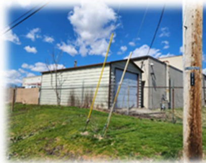
400 N. Erie Blvd P6431050000081 Business Personal Property - Shed
