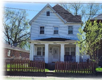
1017 Heaton Street P6431035000007/08 Residential
