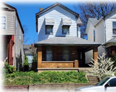
934 Heaton Street P6431025000069 Residential
