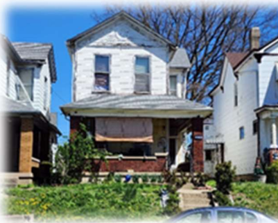
936 Heaton Street P6431025000070 Residential
