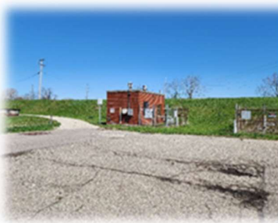
700/1150 Joe Nuxhall Blvd. P6431013000013 Personal Property - Inside Building
