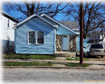
656 Heaton Street P6431017000050 Residential
