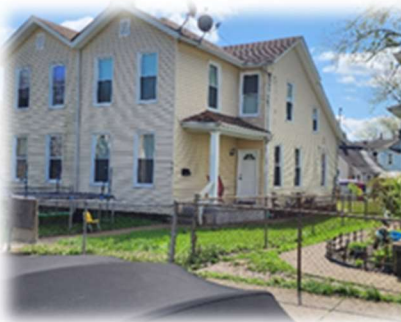
847/849 Greenwood Avenue P6431024000011/12 Personal Property– Shed
