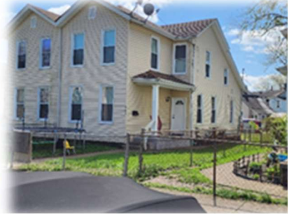
847/849 Greenwood Avenue P6431024000011/12 Personal Property – Shed
