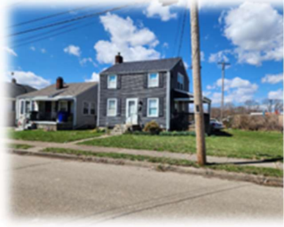
249 Bond Avenue P6431054000006 Residential
