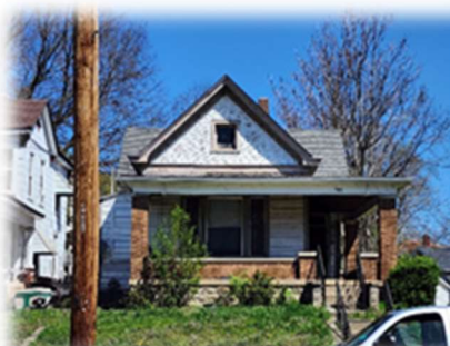
946 Heaton Street P6431025000072 Residential
