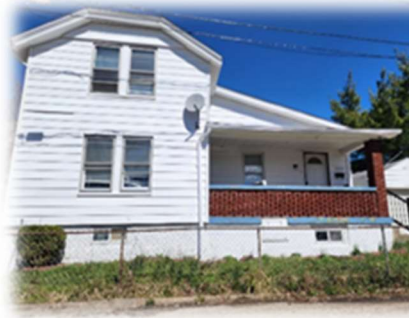
1234 Gilmore Avenue P6431052000024/22 Residential
