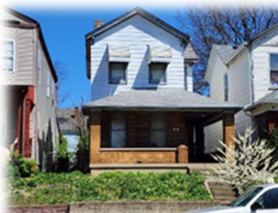
934 Heaton Street P6431025000069 Residential
