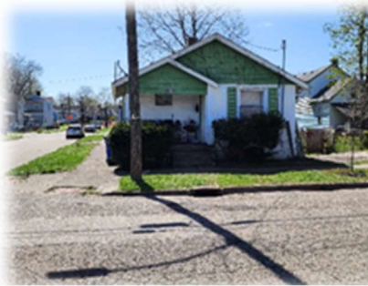
855 Reservoir Street P6431022000029 Residential
