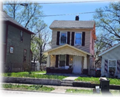
1013 Heaton Street P6431035000004 Residential
