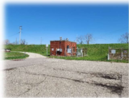
700/1150 Joe Nuxhall Blvd. P6431013000013 Personal Property – Inside Building
