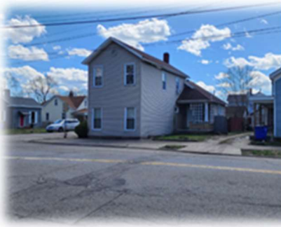
1039 Heaton Street P6431035000014 Residential
