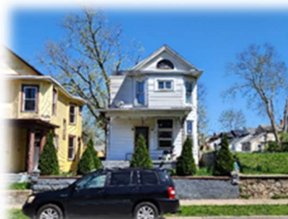
920 Heaton Street P6431025000066 Residential
