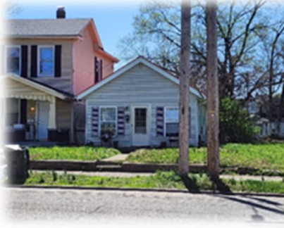
1011 Heaton Street P6431035000003 Residential
