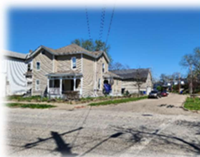
848/850 Heaton Street P6431024000022 Residential – Three-Family including Garage
