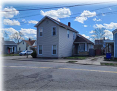
1039 Heaton Street P6431035000014 Residential
