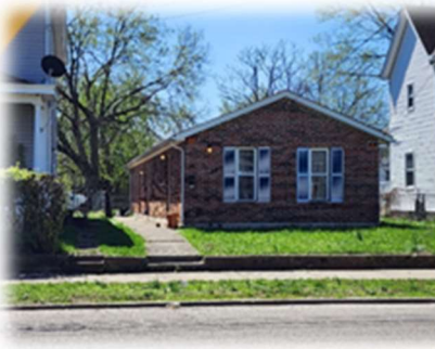
1025 Heaton Street P6431035000009 Residential
