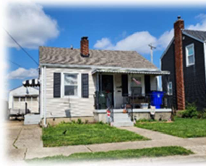
247 Bond Avenue P6431054000007 Residential
