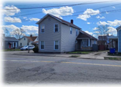
1039 Heaton Street P6431035000014 Residential
