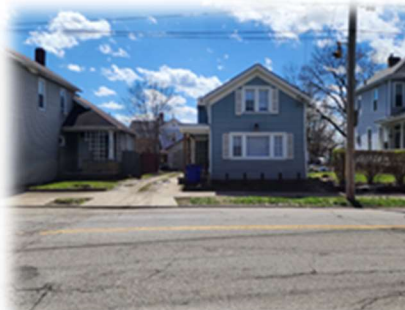
1035 Heaton Street P6431035000013 Residential
