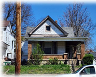
946 Heaton Street P6431025000072 Residential
