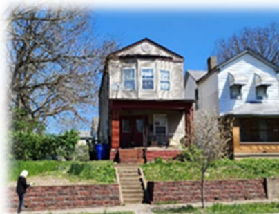
932 Heaton Street P6431025000068 Residential
