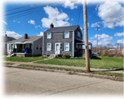
249 Bond Avenue P6431054000006 Residential
