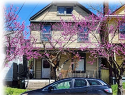
912 Heaton Street P6431025000063 Residential
