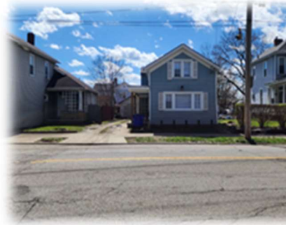
1035 Heaton Street P6431035000013/11 Residential Garage Law may apply
