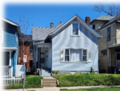
906 Heaton Street P6431025000060 Residential
