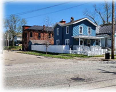
902 Heaton Street P6431025000059 Residential
