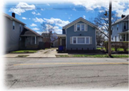
1035 Heaton Street P6431035000011/13a/? Residential
