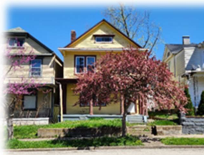
916 Heaton Street P6431025000064 Residential
