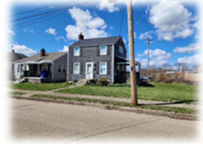
249 Bond Avenue P6431054000006 Residential
