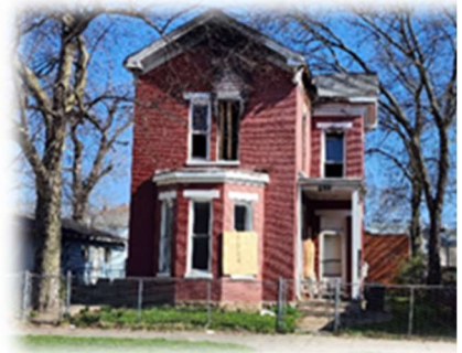
644 Heaton Street P6431017000044 Residential
