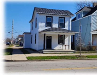
630 Heaton Street P6431017000041 Residential
