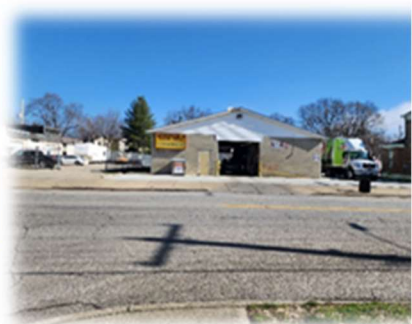
810 Heaton Street P6431024000031 Business (Minnicks) Circuitry issues
