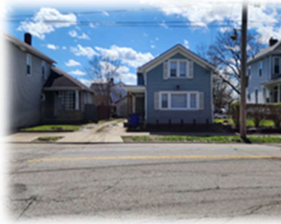
1035 Heaton Street P6431035000013 Residential
