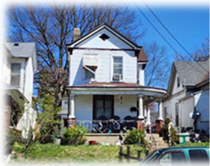
938 Heaton Street P6431025000071 Residential
