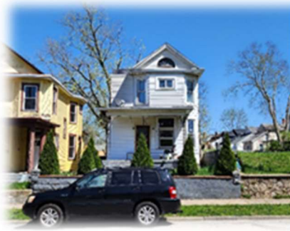
920 Heaton Street P6431025000066 Residential
