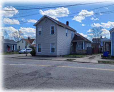
1039 Heaton Street P6431035000046 Residential Garage Law may apply
