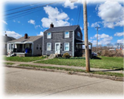
249 Bond Avenue P6431054000006 Residential
