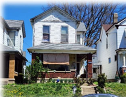
936 Heaton Street P6431025000070 Residential
