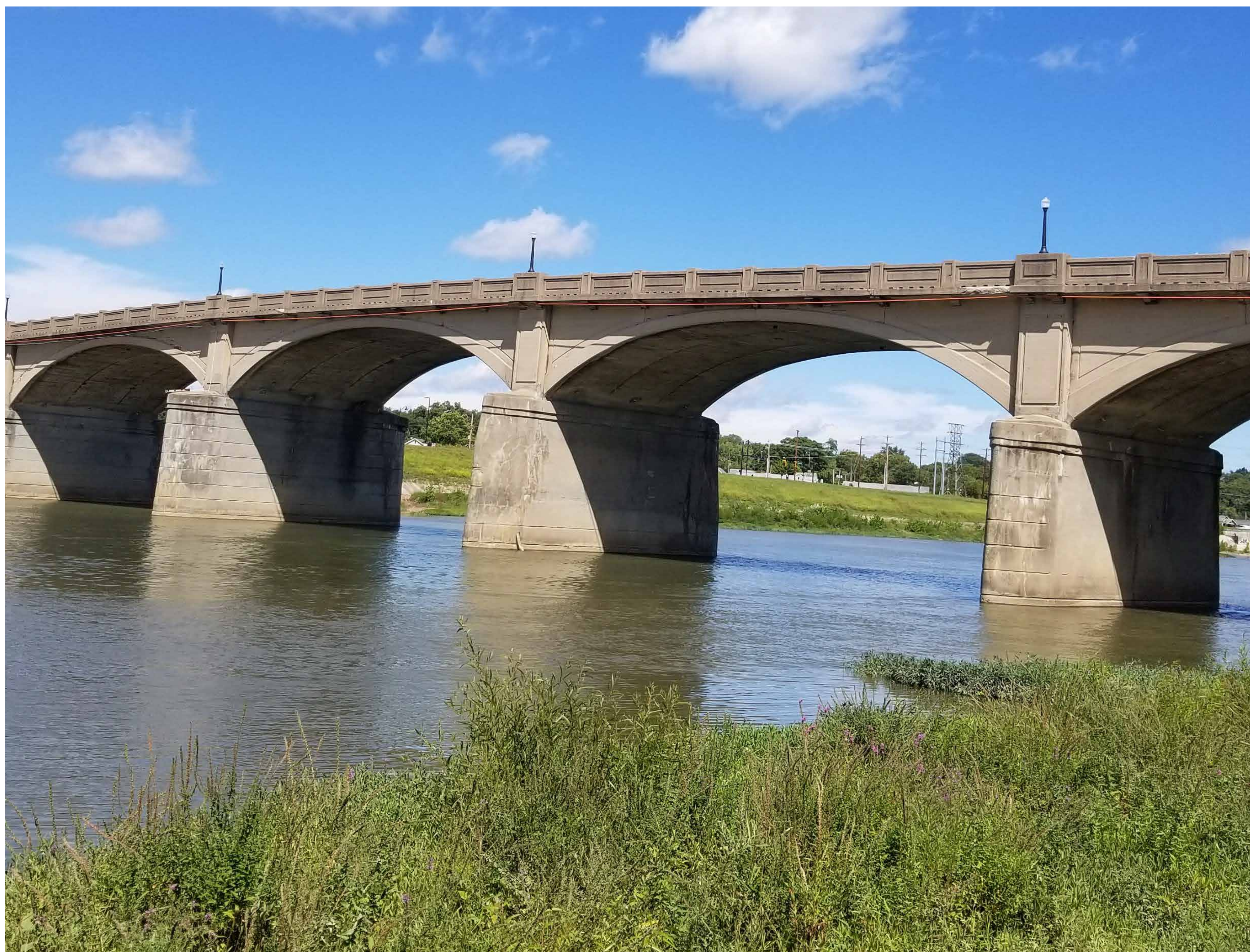
Black Street Bridge
